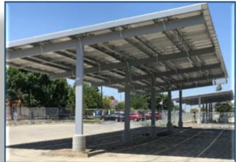
Solar Photovoltaic System Project: Woodland CC
