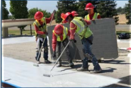
Roof Project, Bld. 100A New Roof Coating: Yuba College
