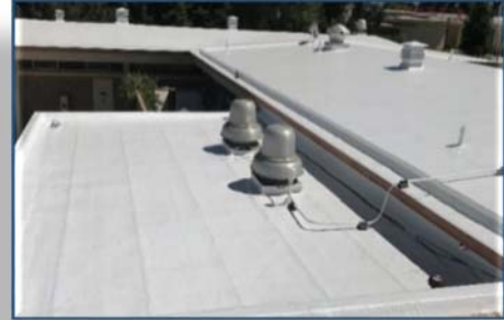
Roof Project, Bld. 500: Yuba College
